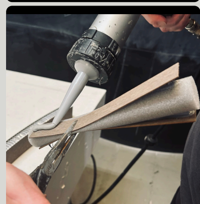
Add the last laminate stick (the one without adhesive)
